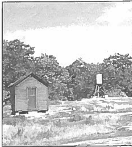
Generator Shed and Water Tower
