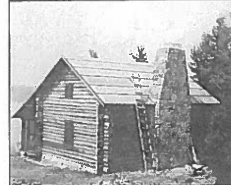
Stone fireplace built by George Washington Brown
